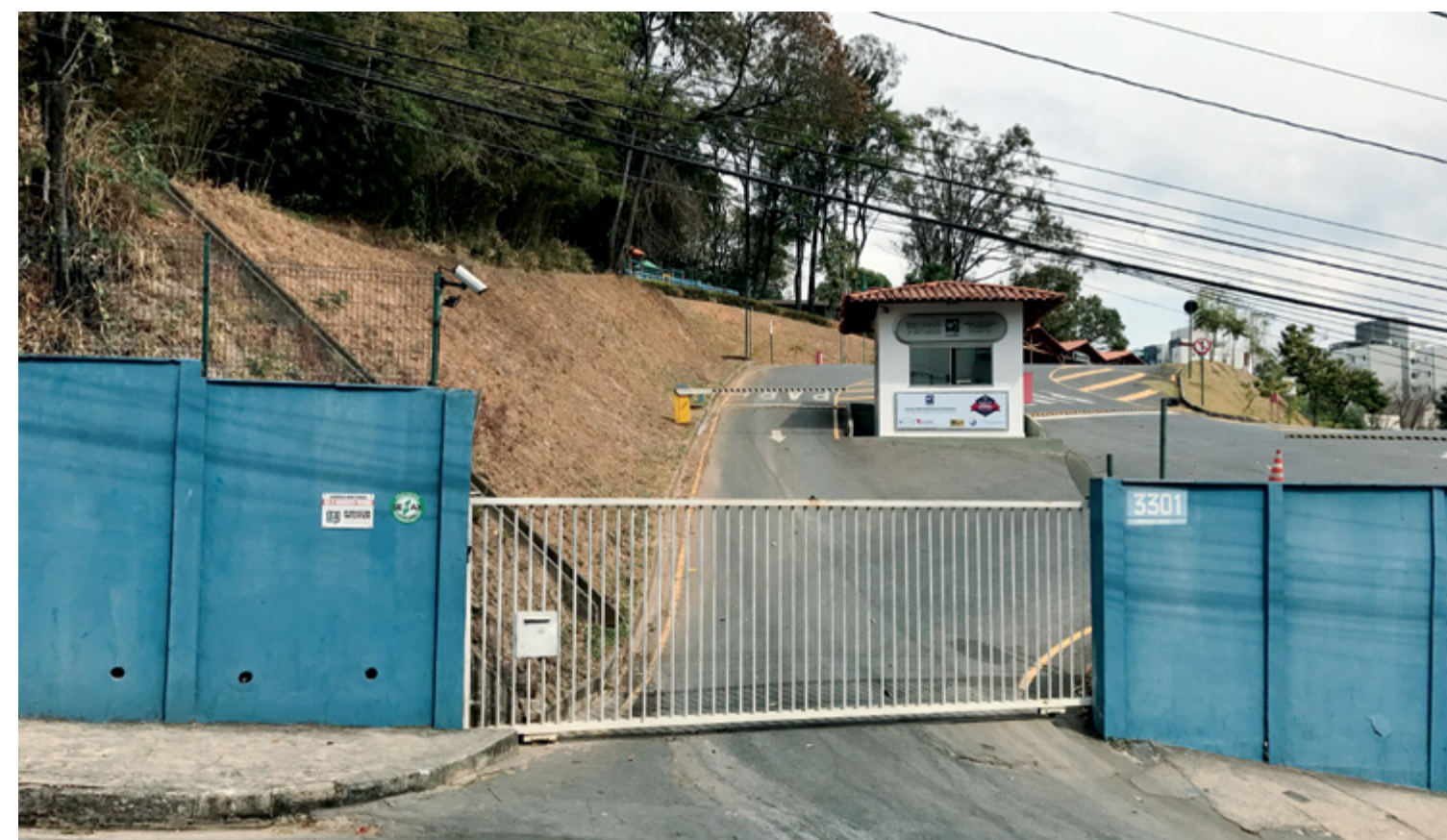
Nova entrada da EABH EABH's new entrance.
